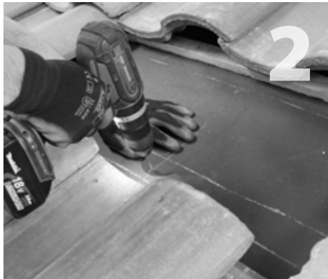
2 Rest the base plate (item 1) over center of rafter and mark center of holes. Drill two 7/32" pilot holes and fill with sealant compatible with roofing materials.
