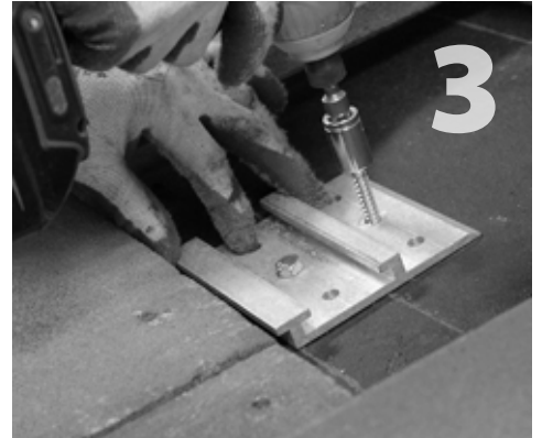
3 Drive lag screws into rafter through the two holes to a solid, snug fit. DO NOT over tighten lag screws, this may compromise their holding strength.
