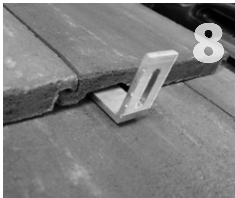
8 Bolt the side-mounted rail of your choice to the hook, using the rail manufacturer's hardware.
