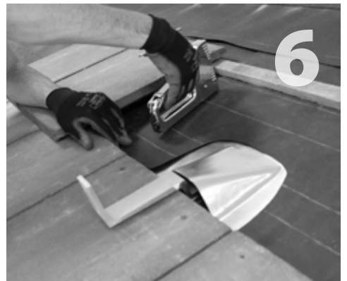
6 Proceed with weatherproofing using three-course method or lapped paper method.* When using paper method, cut a piece of underlayment 18" wide to slide under the course above and over the sub-flashing. If course above is too high, you must use additional underlayment to ensure proper overlapping.
