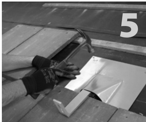
5 Carefully clean the underlayment, then apply bead of compatible sealant in the shape of an upside down U on the backside of the sub-flashing and install flashing over mount. Fasten sub-flashing to deck with one roofing nail in each top corner. Do not nail bottom corners.
