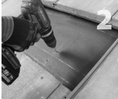
2 Rest the base plate over center of rafter and mark center of holes. Drill two 7/32" pilot holes and fill with sealant compatible with roofing material.
